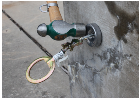
Tap the collar with hammer to align chocks
