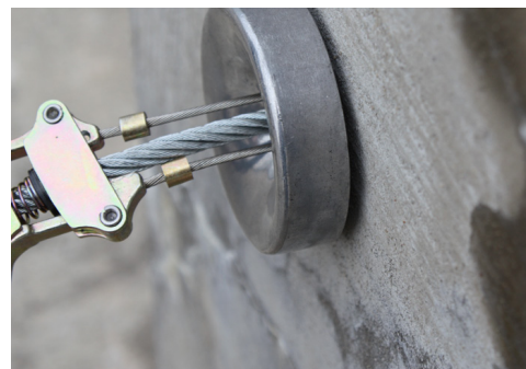
Incorrect Insertion - Collar is NOT flush on concrete
