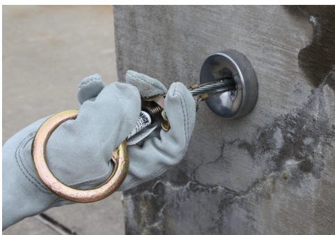
Correct Insertion - Collar is flush on concrete
