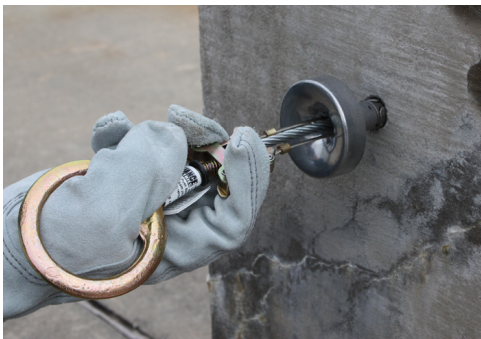
Correct Insertion - Trigger Block is level
