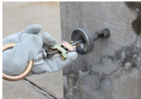
Inorrect Insertion - Trigger Block is NOT level
